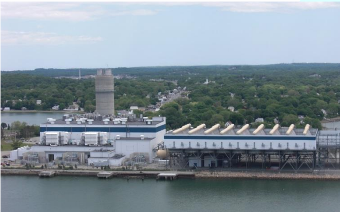
Fore River Energy Center – Weymouth Massachusetts
