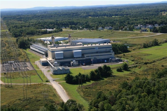
Westbrook Energy Center – Westbrook Maine
